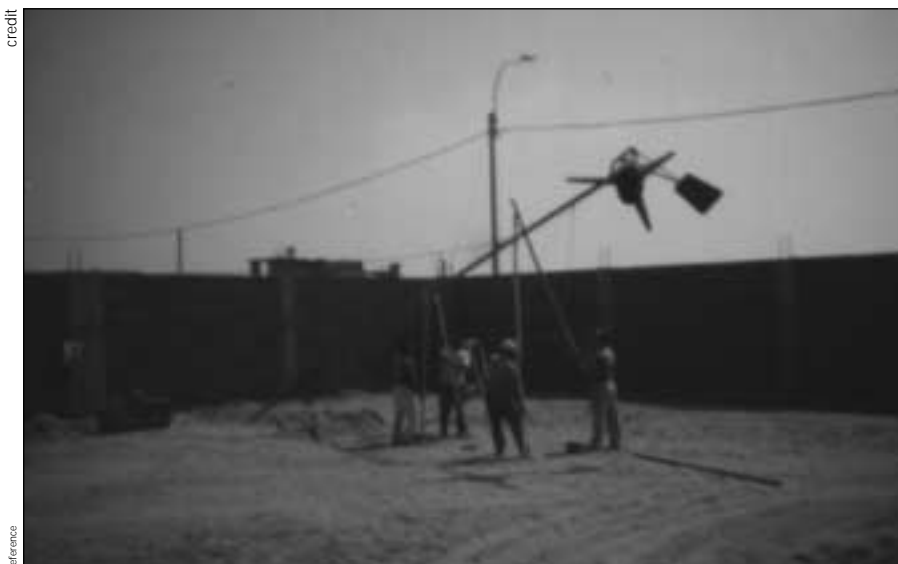
Figure 3: Erecting towers is not as simple as it looks
