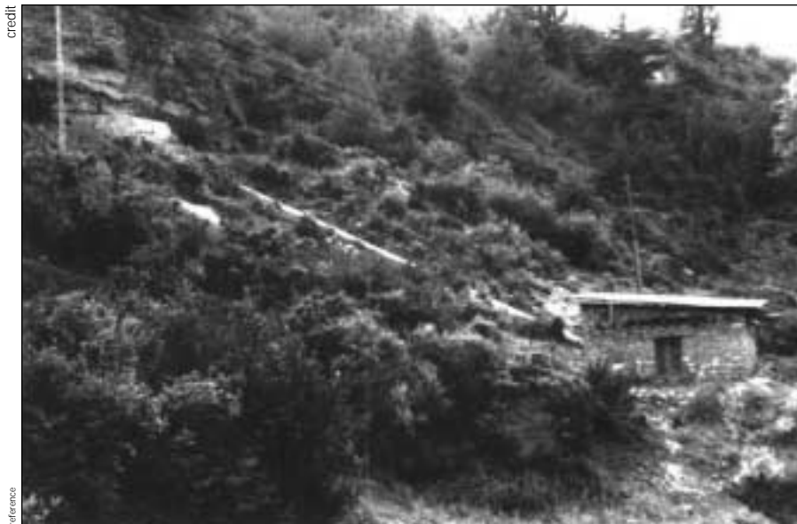
Figure 2: 10kW micro-hydro power system
