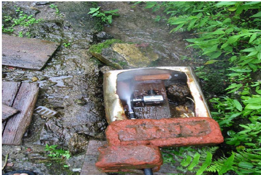
Fig. 12 Pico Hydro (6 Watt, 12 Volt Bicycle Dynamo) in operation in Mamring, India
