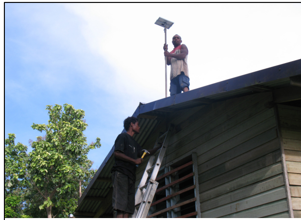
* The installation team works on putting up the solar panel at the rural health facility on Kiriwina Island.
