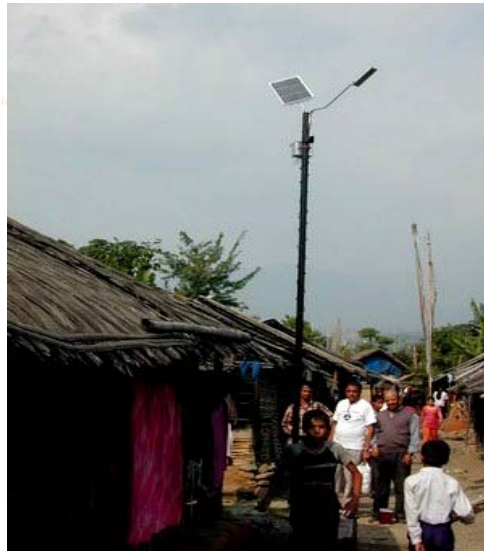
Figure 5 – Solid state street lighting system project in UNHCR refugee camp, Damak, Nepal (2007)
